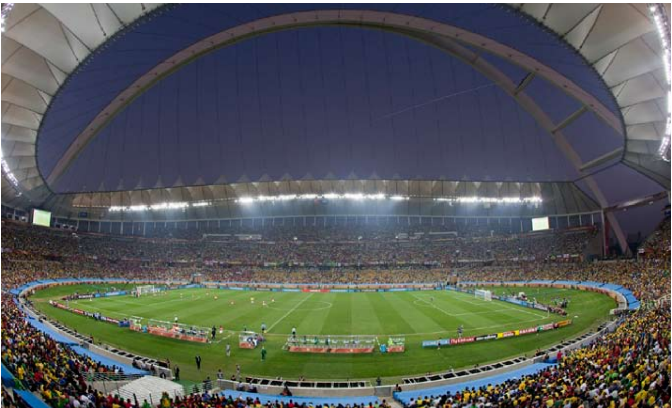
TOP AND BELOW: Moses Mabhida Stadium incorporates the latest in hi-tech and sustainable lighting. The arch overhead is made up of 1.8m LED strip lights, which are 70% more efficient than fluorescent alternatives.
